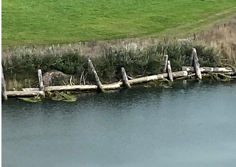
Example biotechnical bank stabilization, with willows and log structures, along a tidally-influenced channel.
